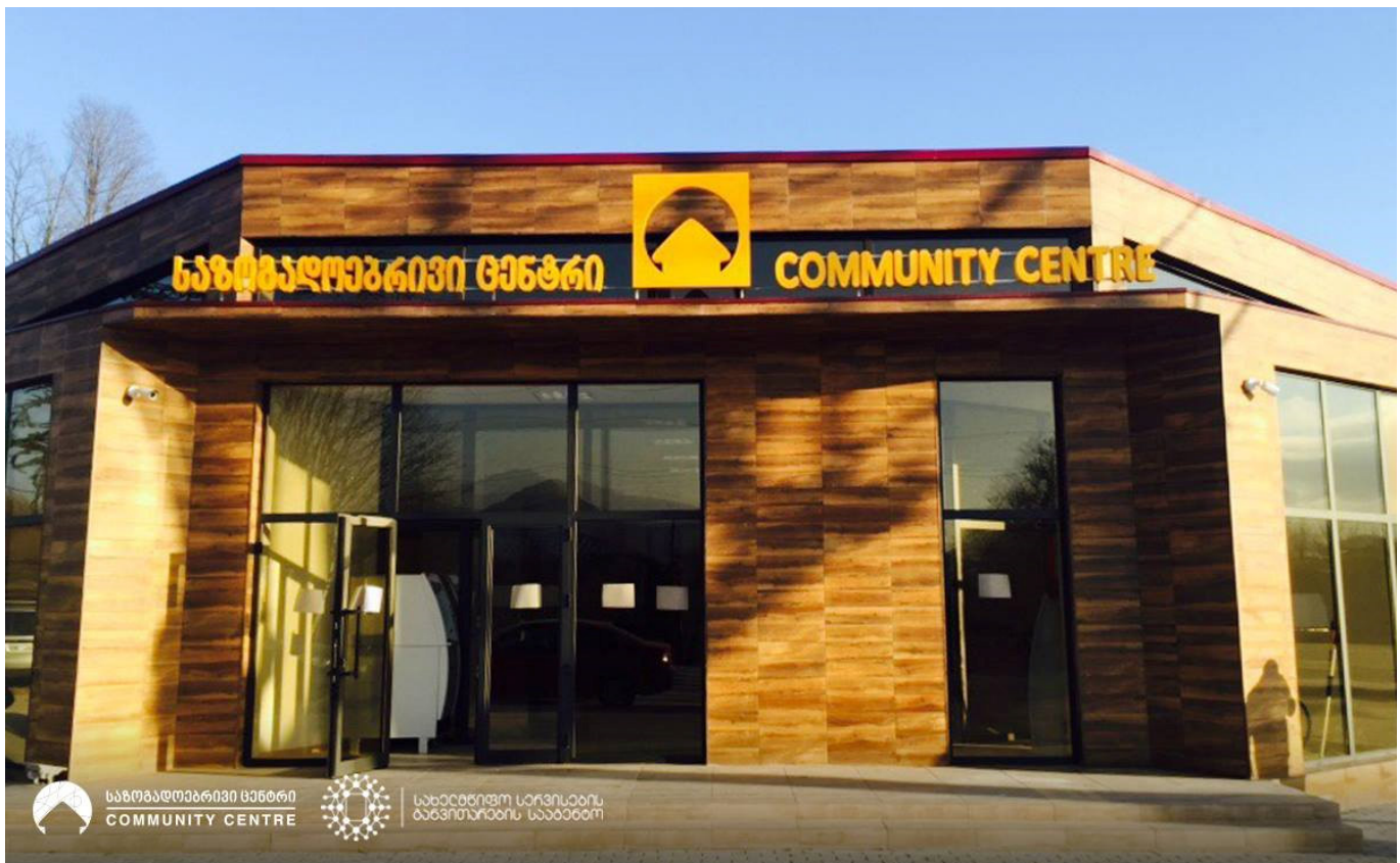
Picture 7 - Community Centre in Georgia
